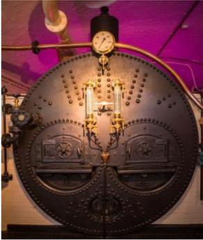
These created steam by burning coal and boiling the water. Each boiler has 2 fires and these fires were burning 24 hours a day.
