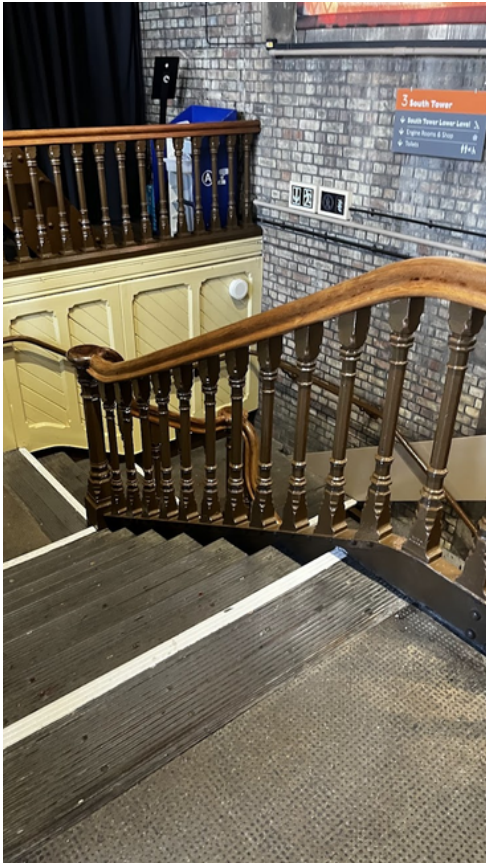
South Staircase (approximately 200 steps)
